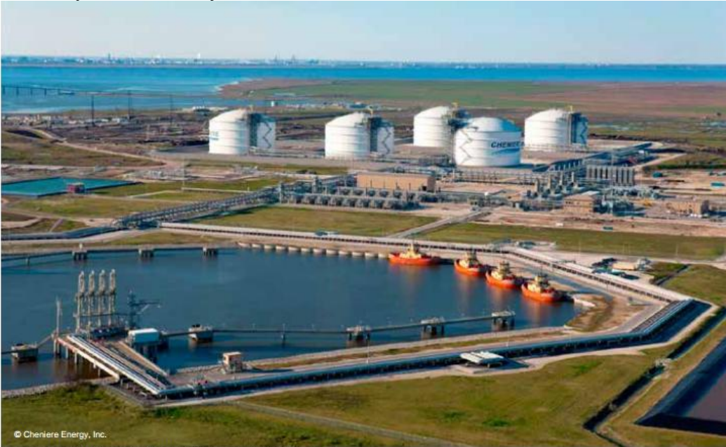
© Cheniere Energy, Inc. Sabine Pass LNG Regasification Terminal, Louisiana, USA
