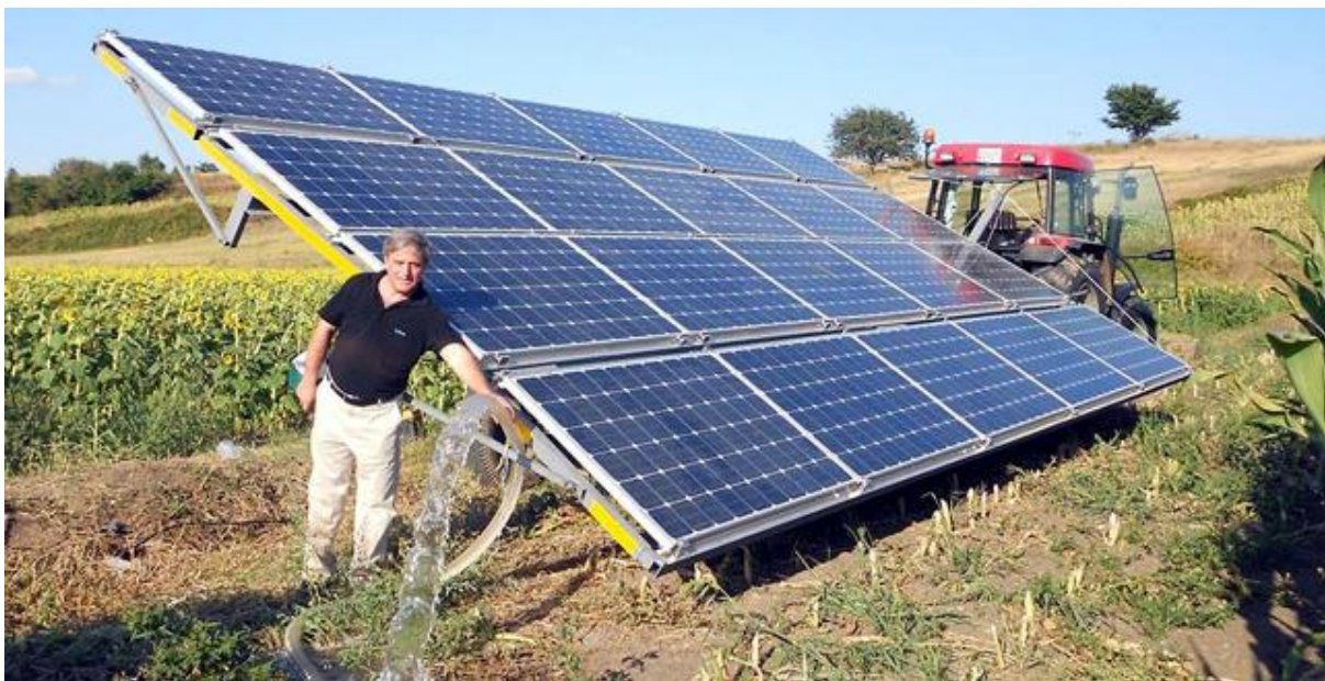
Figure 18. Mobile Solar Powered irrigation system
