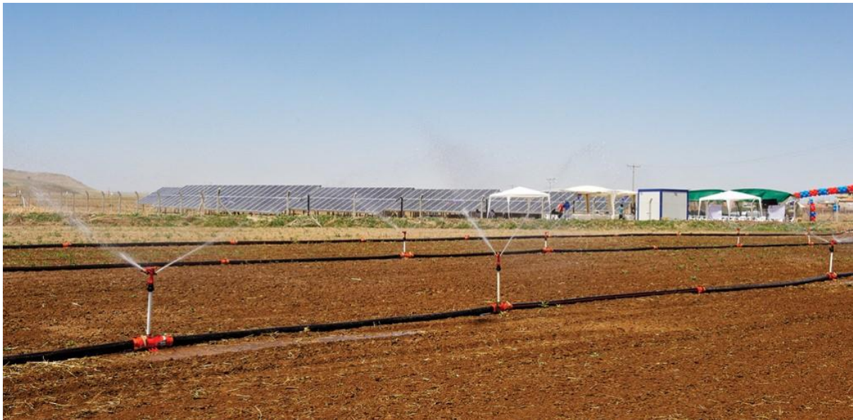
Figure 17. Solar Powered sprinkler irrigation in Turkey.
